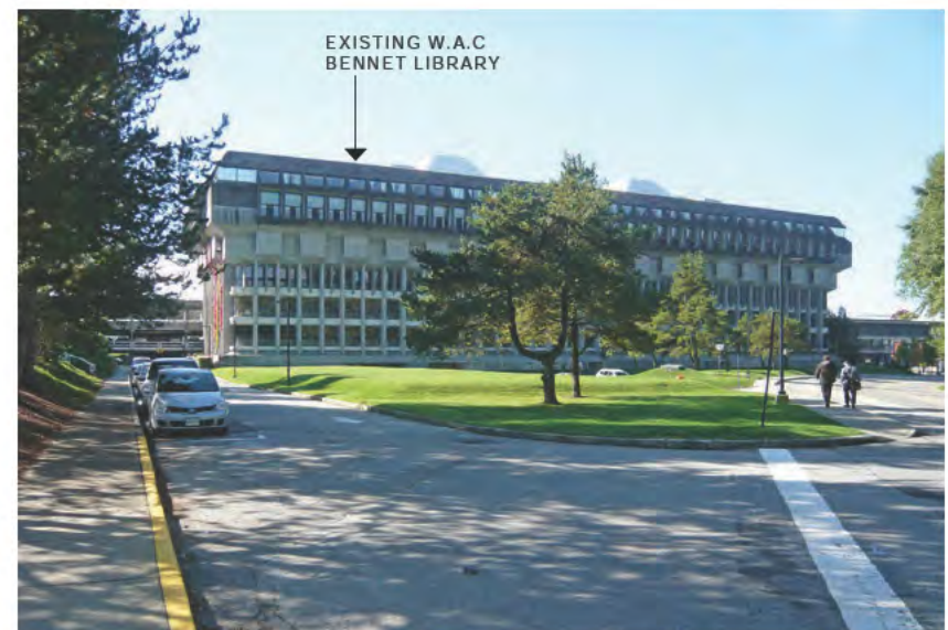
'Pavillion' Building Site, University Drive to right.
