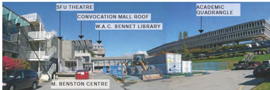
Existing Site Area 3 Looking North
