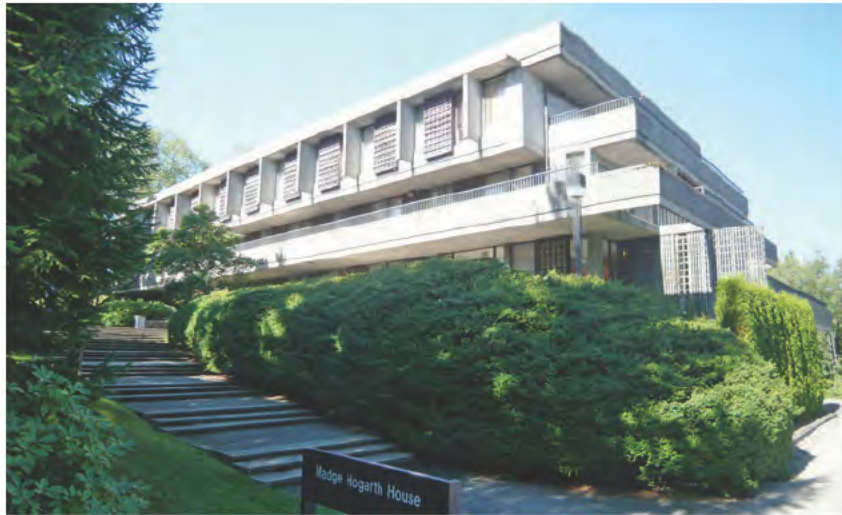
View of Existing Madge Hogarth Building
